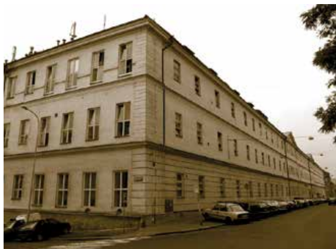
Figure 3. Eye Clinic was located on the second floor in the east wing of the general hospital in Prague (today U Nemocnice 2)
