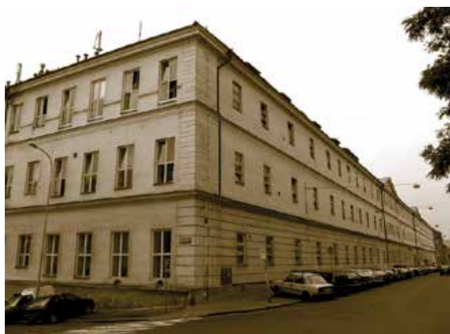
Figure 3. Eye Clinic was located on the second floor in the east wing of the general hospital in Prague (today U Nemocnice 2)
